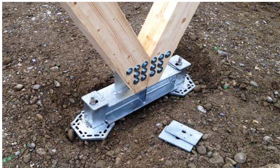
➤ Illustration of a group foundation using steel beams for load distribution or higher individual load absorption.
