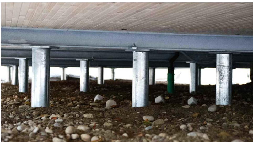
➤ Illustration of a group foundation using steel beams for load distribution or higher individual load absorption.
